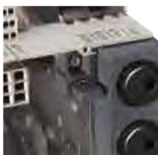
Racking interlock.
