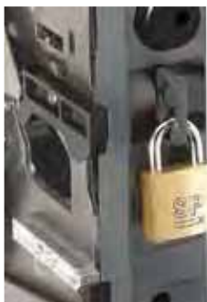
"Disconnected" position locking by padlocks.
